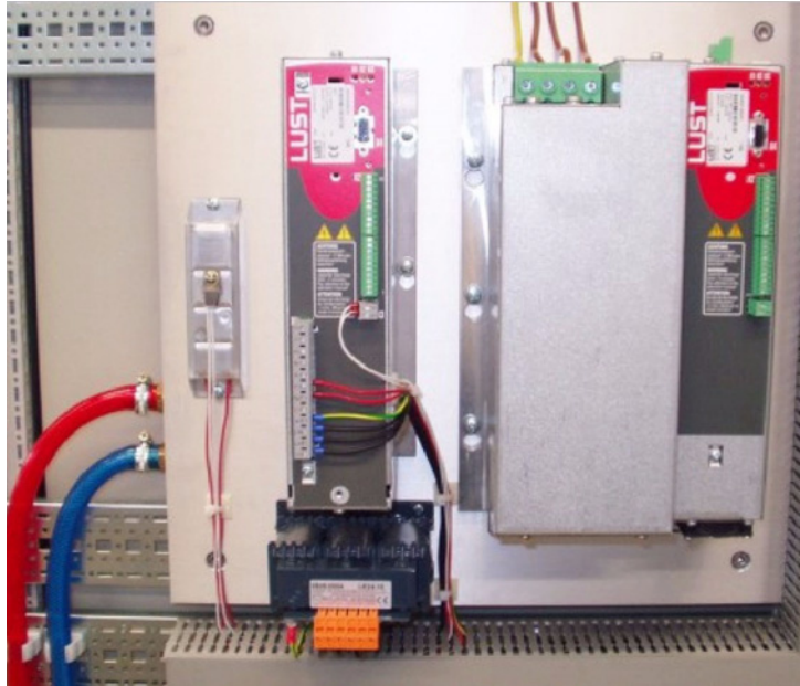
Figure 5.5 Mounting example with CDA3000 and braking resistor on liquid-cooled component backing plate
