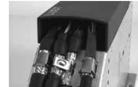
Shield connection with clip and metal cable ties
